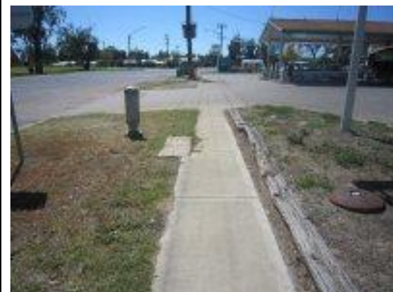
5. A kerb is required to separate the footway from the fuel lanes at Service Stations.
