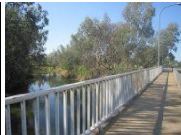
32. Macquarie River Bridge, north side, looking east.
