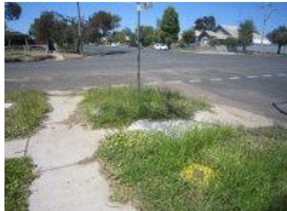
6. Grass overgrowth on footways is a potential trip hazard for people with vision impairment.
