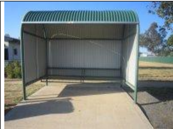
25. TrainLink Bus Stop on the northern side of the Mitchell Highway in Nevertire has no wheelchair space.
