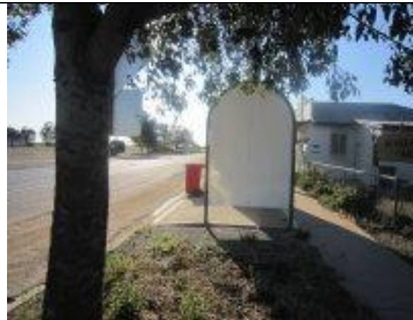
26. TrainLink Bus Stop on the northern side of the Mitchell Highway in Nevertire has a steep Boarding Point and no connecting path to the footway.
