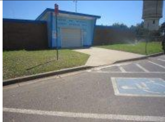
30. A parallel Accessible Parking Space near the entrance to the Pool, just south of the kerb ramp is recommended.
