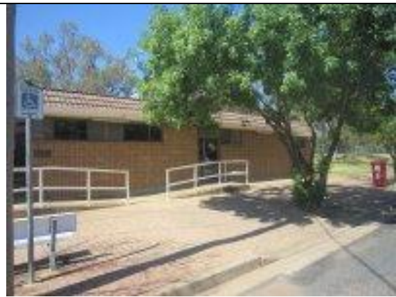
18. Lower rail required.
