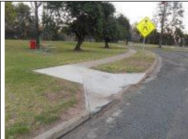
11. Correctly constructed kerb ramp.
