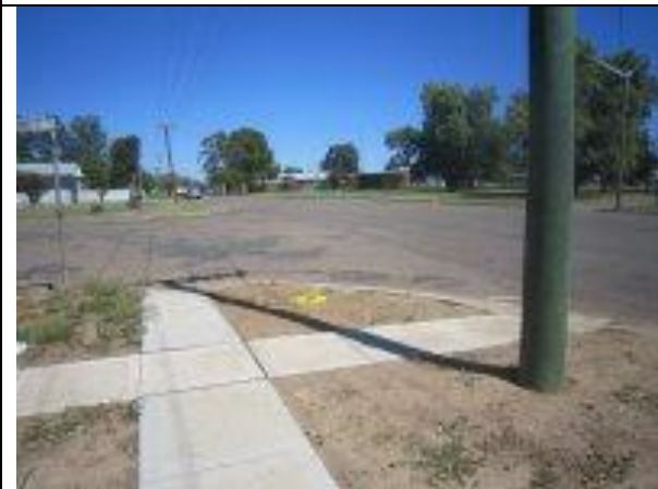
13. Radius kerb needs to be reduced to allow the construction of standard kerb ramps.
