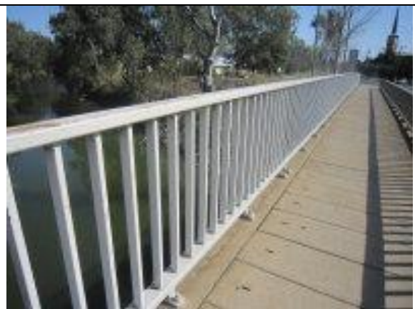
33. Macquarie River Bridge, south side, looking west.
