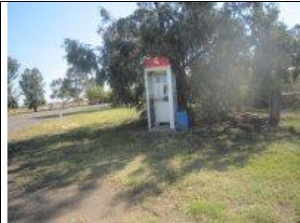
21. Public Telephone is not accessible. A hard-stand area, with circulation space 1540 mm X 2070 mm, is required in front of the door.
