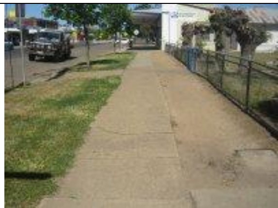
20. The bare surface at the side of the footway is lower than the footway level.
