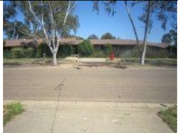
16. A walk-through at the same level as the roadway would assist people who use a wheelchair. TGSIs are required.
